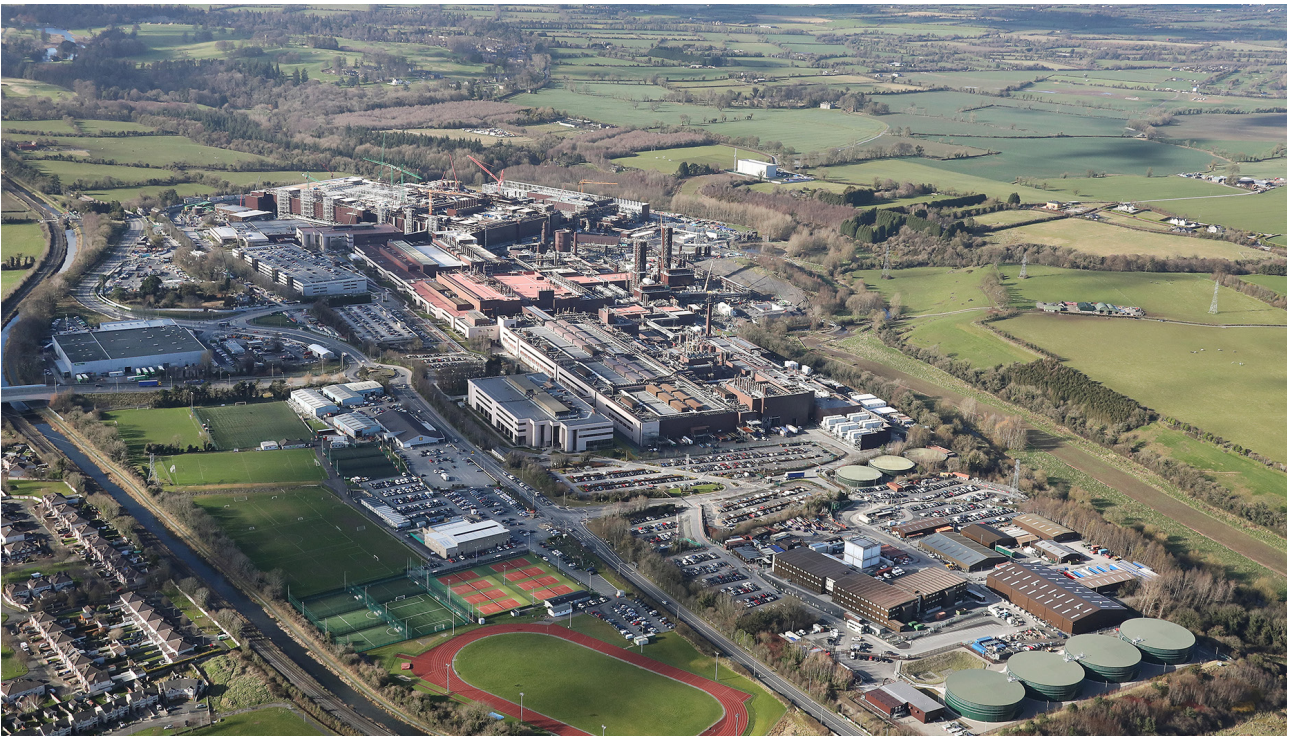
Aerial photo of the Intel Leixlip campus in Ireland.
